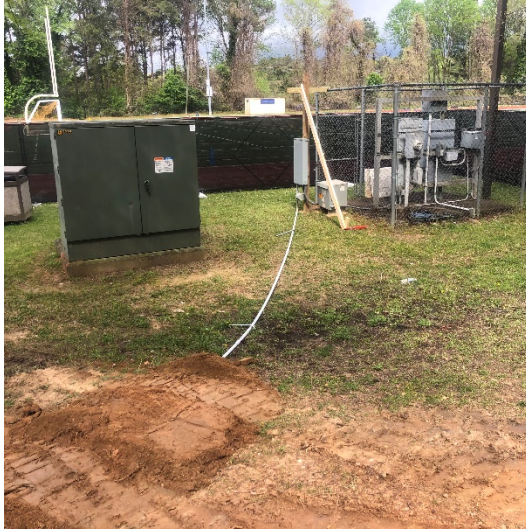
Temporary Power Installed
